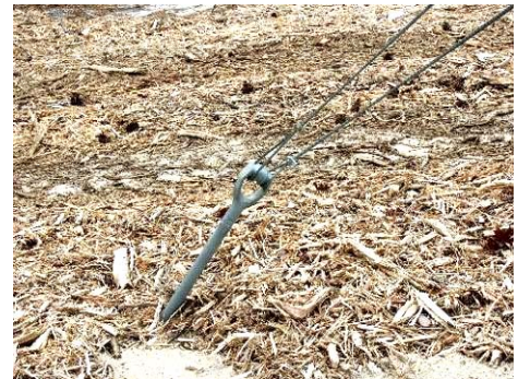
An anchor, installed, with 2 guy wires attached
